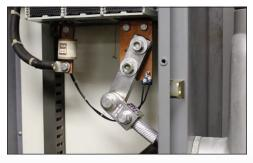
ROTO-LUG™ connectors allow for the wire to be landed in a straight line in a switchgear box or breaker.
